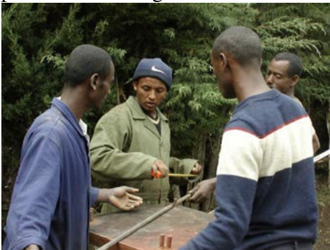
Bending rebar in Ethiopia
