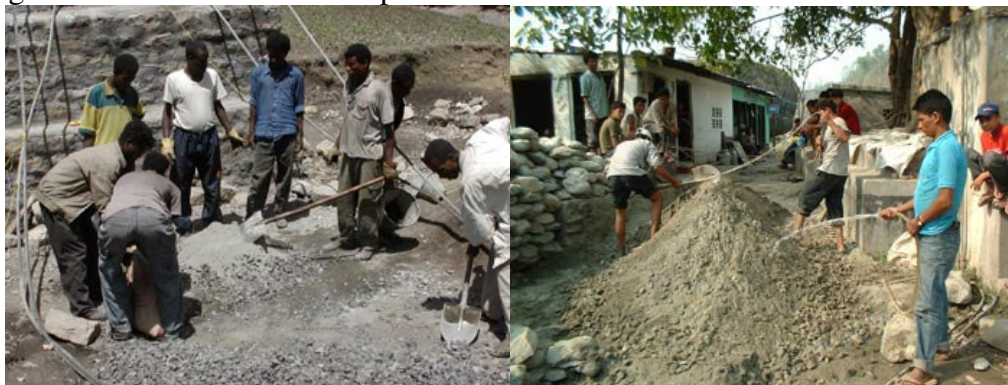
Mixing the dry materials
