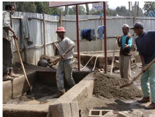
Washing sand at an industrial site
