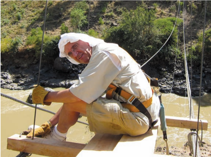
Bill at work on the bridge (Photo: Brett Hargrave)
