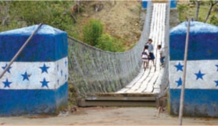
Children play on their new bridge at Mezcalillo, Honduras
