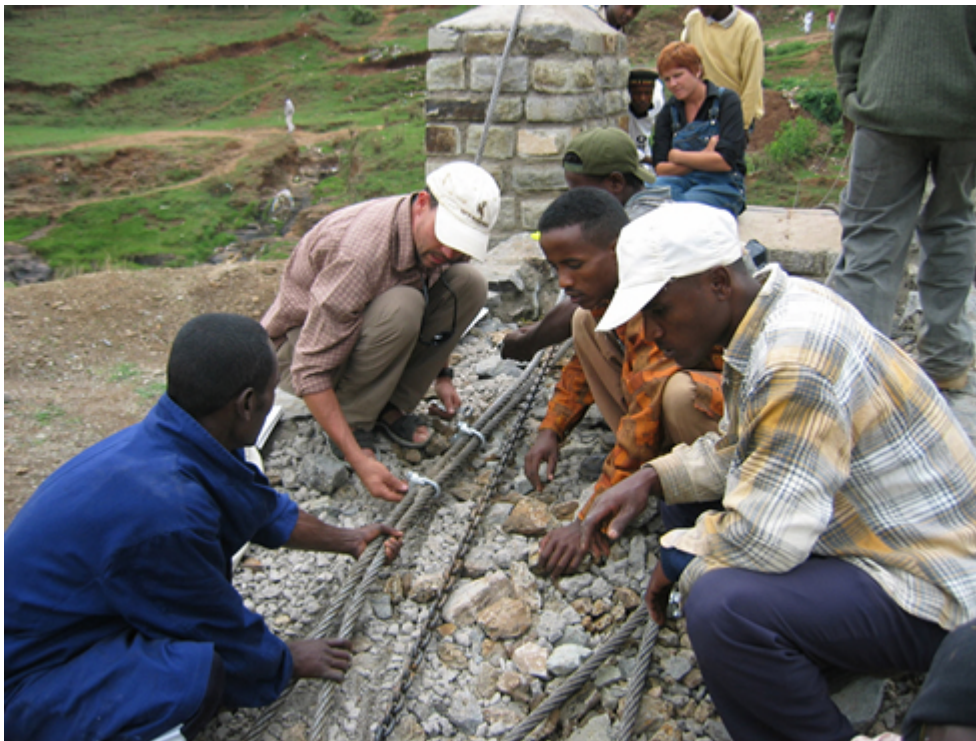
Preparing to set the sag on the cables (Richard James Photography)
